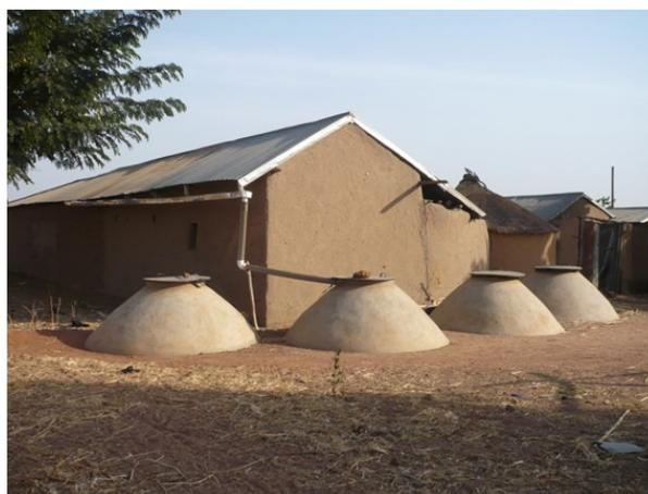
**Fig. 1 Rooftop rainwater harvesting system with interconnected ferrocement tanks**
