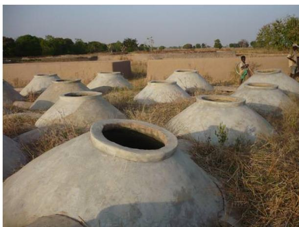
**Fig. 2 Stream flow collection in interconnected ferrocement tanks**
