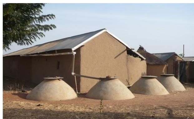
Fig.4: Rooftop rainwater harvesting system with interconnected ferro-crete tanks
